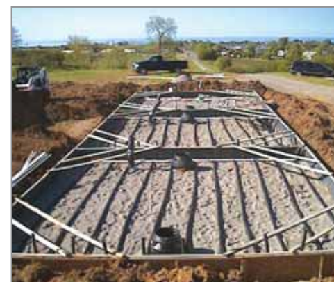
Left: A three-cell vertical wetland under construction, including pump chambers, perforated collection pipes and a 30-mil PVC liner that is flexible for easy installation and pliable in cold weather. Center: The vertical wetland components are covered with filtering media, which varies depending on treatment objectives and wastewater characteristics (i.e., particle size, porosity and aluminum, iron and calcium content) and treatment objectives. Right: The vertical wetland is planted with cattails (Typha sp.) or reed grass (Phragmites sp.), again depending on wastewater characteristics (Phragmites, for example are more tolerant of high ammonia concentrations).
